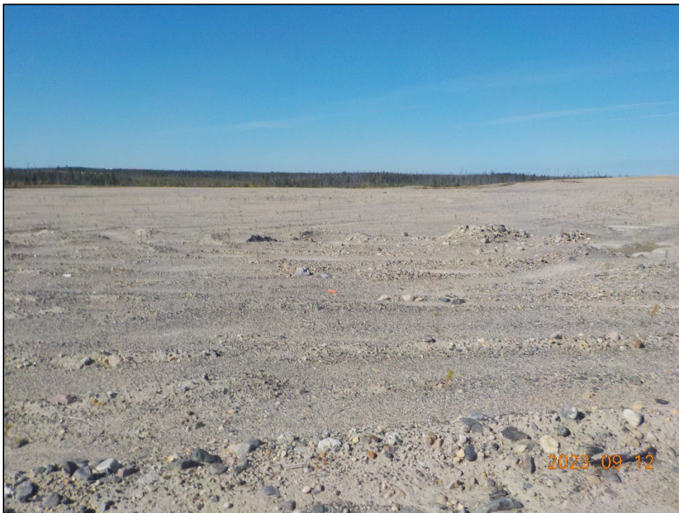
Photo 4-2: Barren vegetation cover and structure in Borrow Area G-3.
