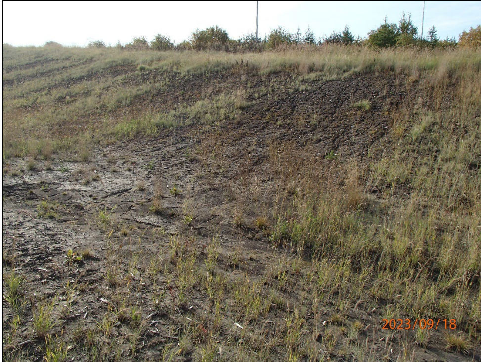
Photo 4-11: Regenerating seeded slope with vegetation gaps at an area surveyed for poor regeneration along the North Access Road in 2023
