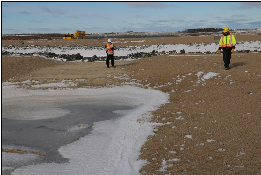
Photo 5-11: Pre-impoundment construction of colonial waterbird Habitat Compensation Island, 2019
