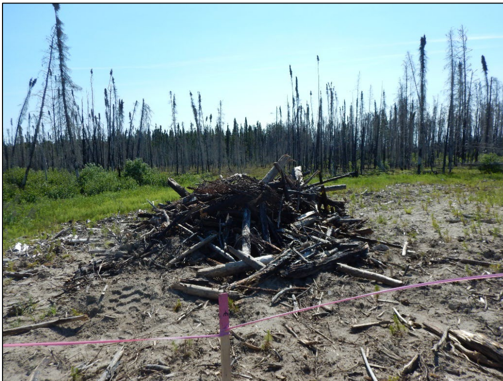
Photo 4-2: Slash pile for amphibian habitat enhancement in KM-4 borrow area, 2017
