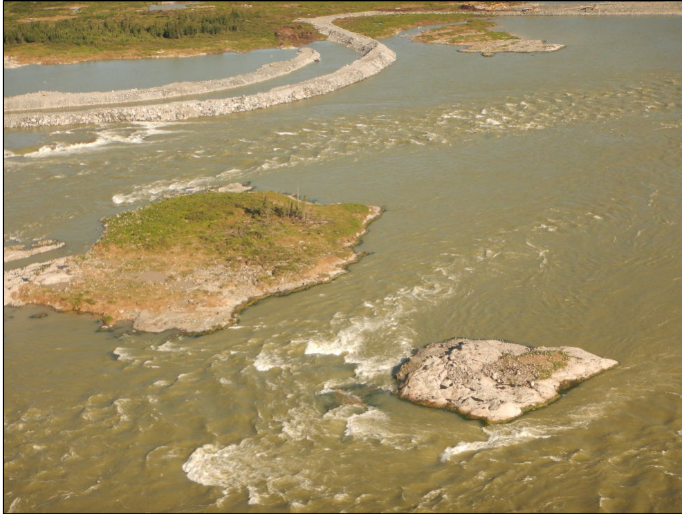
Photo 5-12: Colonial waterbird nesting islands in Gull Rapids, 2015. (Note Project cofferdam construction in background.)
