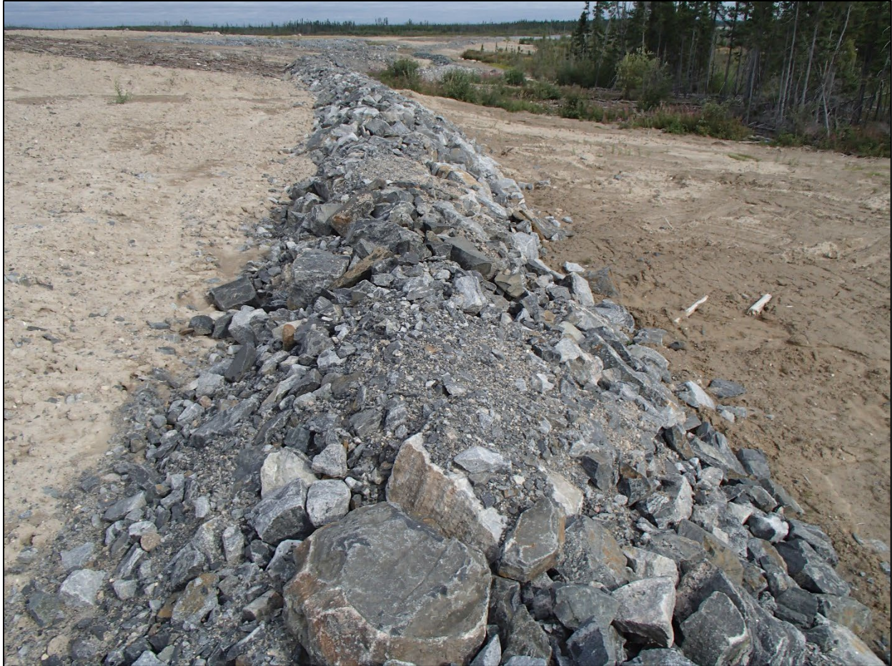
Photo 2-6: Rock berm around EMPA D16(1)-E in 2019
