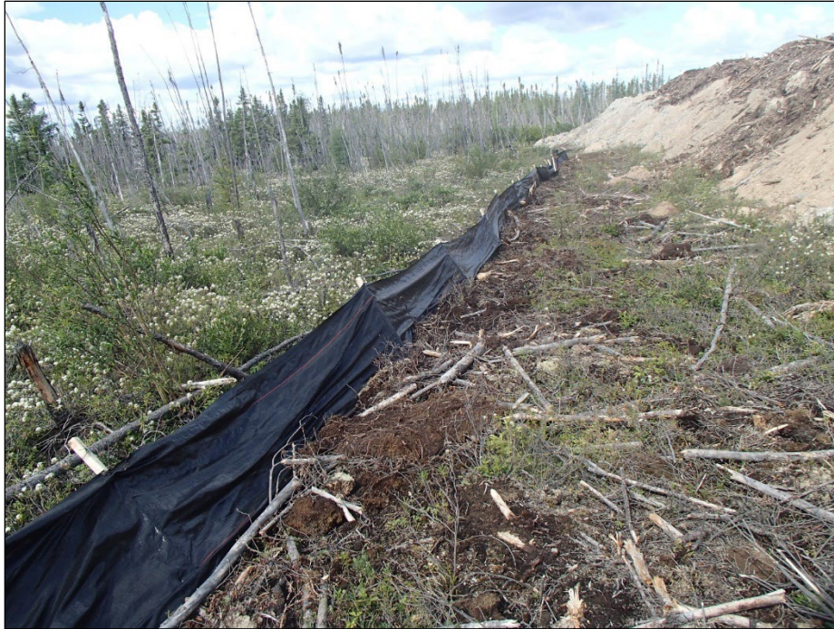
Photo 2-4: Sediment fence deployed after terrestrial habitat survey
