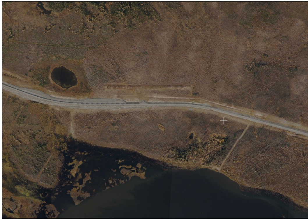
Photo 2-25: Example stereo photo of new cutlines and dike north of Gull Lake used for the Project features mapping
