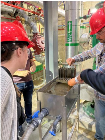
Zebra mussels are in the Nelson River, so they are also found at Keeyask. Because we can't see inside the pipes at Keeyask, we use bio-boxes to check for zebra mussel growth. These bio-boxes tell us when we need to use chlorine to kill the zebra mussels and stop the pipes from getting clogged. This treatment happens once the bio-boxes show the mussel growth in the pipes is too high.
