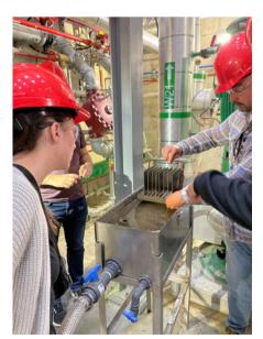
Zebra mussels are in the Nelson River, so they are also found at Keeyask. Because we can't see inside the pipes at Keeyask, we use bio-boxes to check for zebra mussel growth. These bio-boxes tell us when we need to use chlorine to kill the zebra mussels and stop the pipes from getting clogged. This treatment happens once the bio-boxes show the mussel growth in the pipes is too high.
